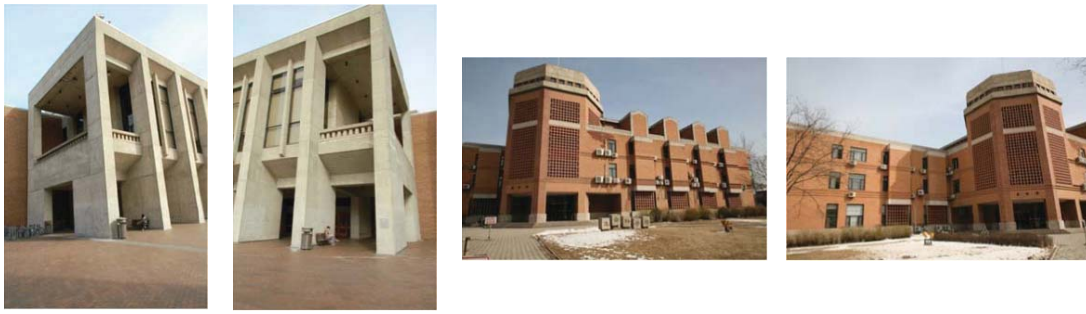
Fig. 14. Sample images of the large data sets. The left two images are from Hull and the right two images are from Life Science Building.
